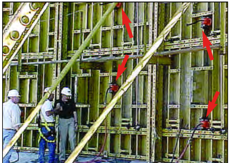
Close up of vibrator spacing.
