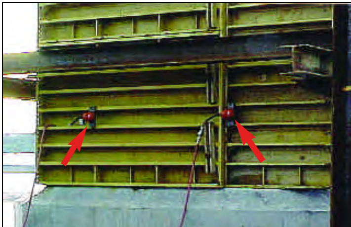
Vibrators placed on 6' centers around form. Next higher row 6' up.
