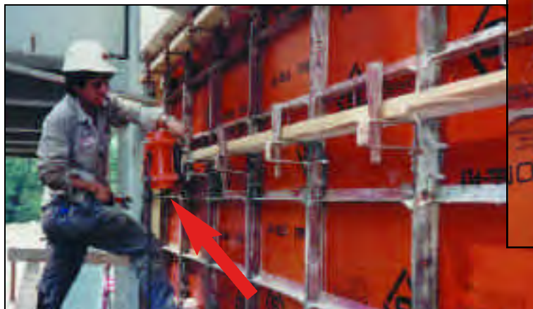
Bracket with vibrator clamped to a 2 x 6.
