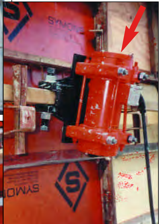
Bracket with vibrator clamped to a 2 x 6.
