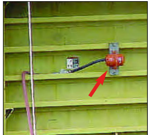
Special Bracket straddling two form stiffeners.
